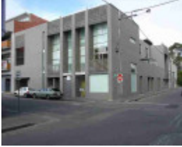
fitzroy st david street fitzroy st david street 30-38
