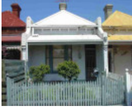
fitzroy north clauscen street fitzroy north clauscen street 138
