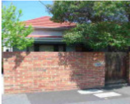
fitzroy north clauscen street fitzroy north clauscen street 142
