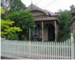
fitzroy north holden street fitzroy north holden street 70
