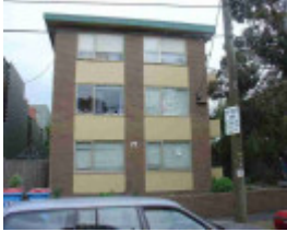
fitzroy north holden street fitzroy north holden street 71
