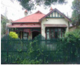
fitzroy north holden street fitzroy north holden street 72
