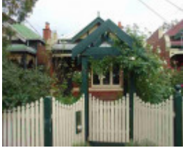
fitzroy north holden street fitzroy north holden street 83
