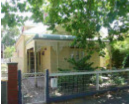
fitzroy north holden street fitzroy north holden street 255
