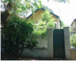
fitzroy north holden street fitzroy north holden street 259
