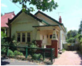
fitzroy north holden street fitzroy north holden street 265
