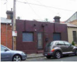
Purfleet Cottages 35-37 Bedford Street
