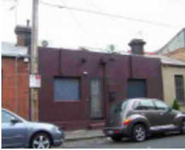
Purfleet Cottages 35-37 Bedford Street
