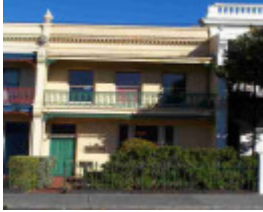
Byrne's Arcade Terrace - 318 Victoria Street
