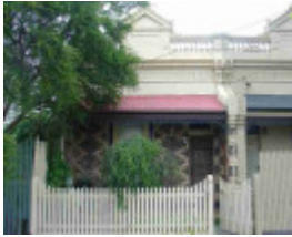
fitzroy north holden street fitzroy north holden street 44
