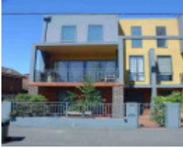
fitzroy north barkly street fitzroy north barkly street 148 unit 1
