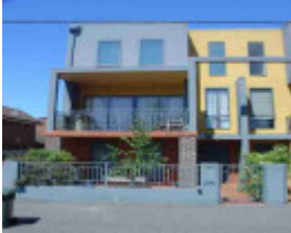
fitzroy north barkly street fitzroy north barkly street 148 unit 3
