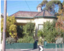
fitzroy north bennett street fitzroy north bennett street 2
