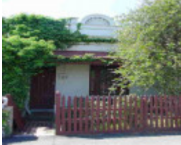
fitzroy north bennett street fitzroy north bennett street 12
