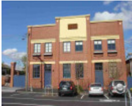
fitzroy north mckean street fitzroy north mckean street 46 unit 1
