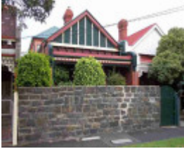
fitzroy north holden street fitzroy north holden street 86
