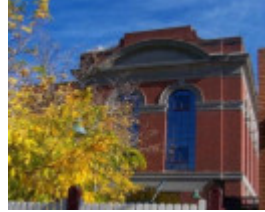
Victorian Railways DC Substation
