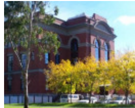
Victorian Railways DC Substation
