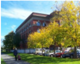
Victorian Railways DC Substation
