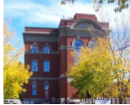
Victorian Railways DC Substation
