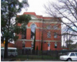
Victorian Railways DC Substation
