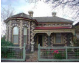
fitzroy north rushall crescent fitzroy north rushall crescent 16
