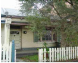
fitzroy north rushall crescent fitzroy north rushall crescent 17
