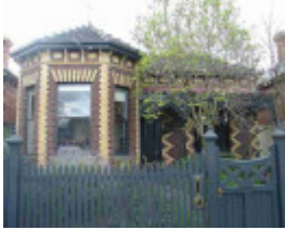
fitzroy north rushall crescent fitzroy north rushall crescent 31
