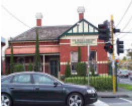
fitzroy north nicholson street fitzroy north nicholson street 842
