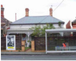
fitzroy north nicholson street fitzroy north nicholson street 844
