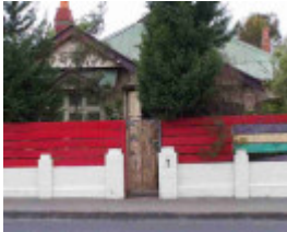
fitzroy north nicholson street fitzroy north nicholson street 860
