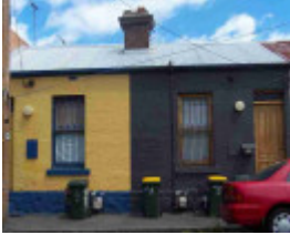
Purfleet Cottages 47 bedford street
