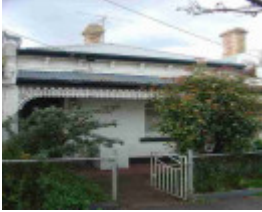
fitzroy north egremont street fitzroy north egremont street 30
