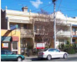
Byrne's Arcade Terrace - 326 Victoria Street
