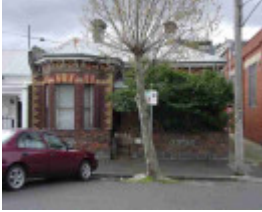
fitzroy kerr street fitzroy kerr street 189
