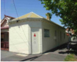
Fitzroy North Rae Street 88.JPG
