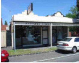
fitzroy north holden street fitzroy north holden street 160
