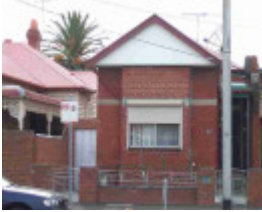
fitzroy north holden street fitzroy north holden street 163
