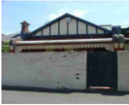
fitzroy north holden street fitzroy north holden street 197
