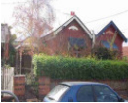
fitzroy north holden street fitzroy north holden street 203
