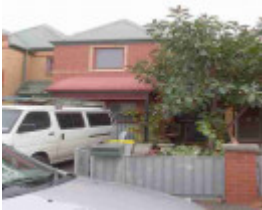
fitzroy north holden court fitzroy north holden court 9
