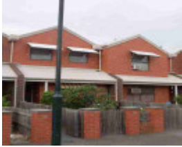
fitzroy north holden court fitzroy north holden court 10
