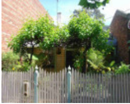
Fitzroy North Rae Street 45.JPG
