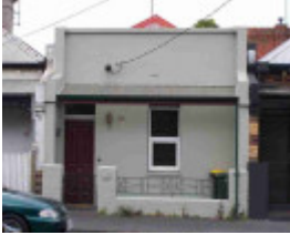
fitzroy north nicholson street fitzroy north nicholson street 874
