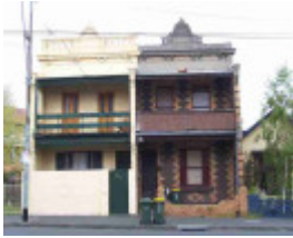
fitzroy north nicholson street fitzroy north nicholson street 882
