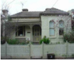
fitzroy north mark street fitzroy north mark street 12
