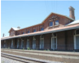
SERVICETON RAILWAY STATION SOHE 2008
