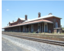
SERVICETON RAILWAY STATION SOHE 2008
