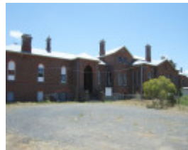
SERVICETON RAILWAY STATION SOHE 2008
