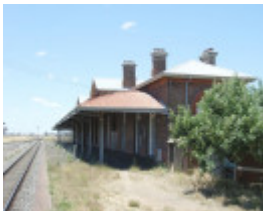
SERVICETON RAILWAY STATION SOHE 2008
