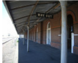
SERVICETON RAILWAY STATION SOHE 2008
