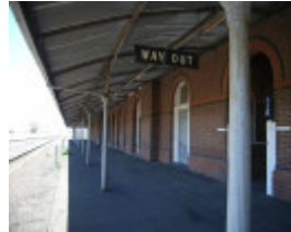
SERVICETON RAILWAY STATION SOHE 2008
