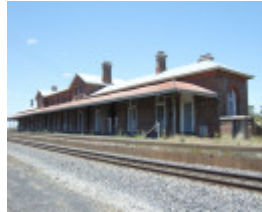
SERVICETON RAILWAY STATION SOHE 2008
