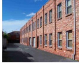
Fitzroy North McKean Street 274.JPG
