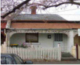
fitzroy north jamieson street fitzroy north jamieson street 2
