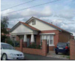
fitzroy north white street fitzroy north white street 6
