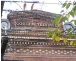
Cobden Terrace - Parapet
