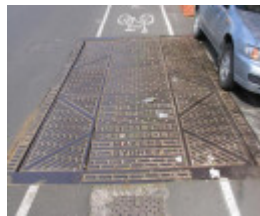
Weighbridge in Oxford Street
