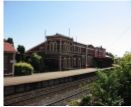
Seymour RWS Railway Building Road Side February 2002
