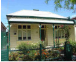
fitzroy north holden street fitzroy north holden street 116
