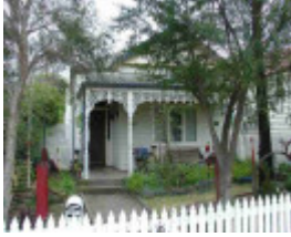
fitzroy north holden street fitzroy north holden street 117
